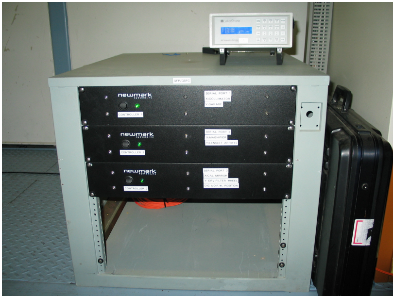
Fig. C.4 GIII components on the Mezzanine Level, with the Lakeshore heater controller sitting on top of the Newmark drive controllers.
