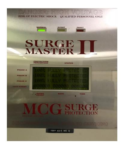
Note: NORMAL is lit in green; FAULT is not lit; Protection is 100% for each of the 3 phases.
