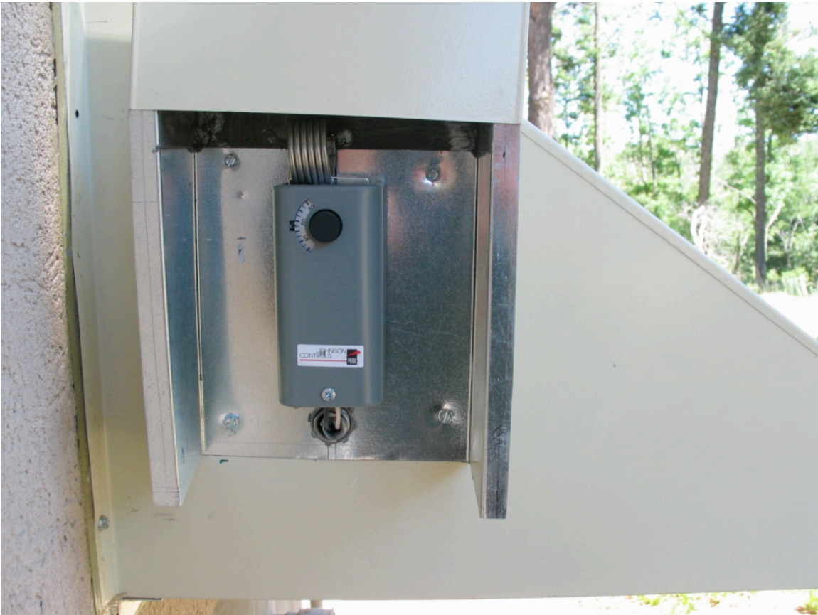
Figure 4 Fresh air inlet louver temperature control
