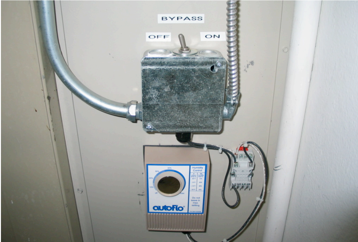
FIGURE 2 Fresh air inlet louver bypass and humidity control
