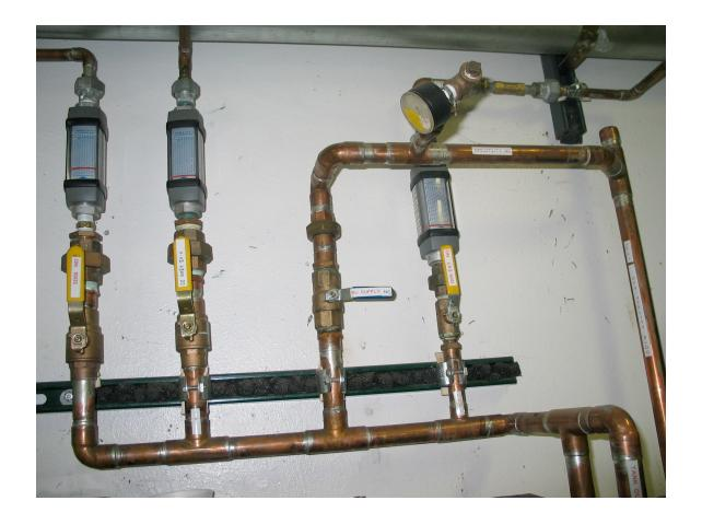
If both dryers mounted on the wall or the filters fail air can be fed directly from the tank to the distribution manifold by closing the outlet valve at the bottom of the tank and opening the outlet valve near the top of the tank as shown in fig 2. This will allow "dirty and wet" air to be distributed and thus should 1. only be used in an emergency and 2. the optic flush lines at the SDSS imager/Spectrograph and SpiCam and Dis for the 3.5m should be closed off.
